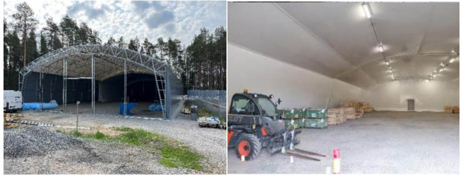
TENT construction and finished article
